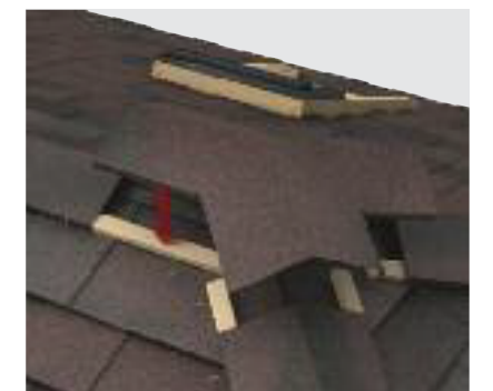
Fix rafter cap and ridge
