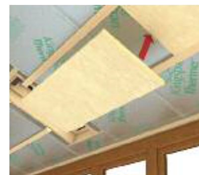
Install insulation between batten
